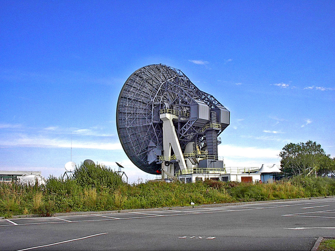
Goonhilly Satellite Earth Station
